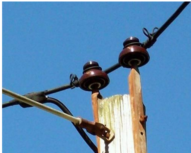
Gambar 2.2 Isolator Pin
