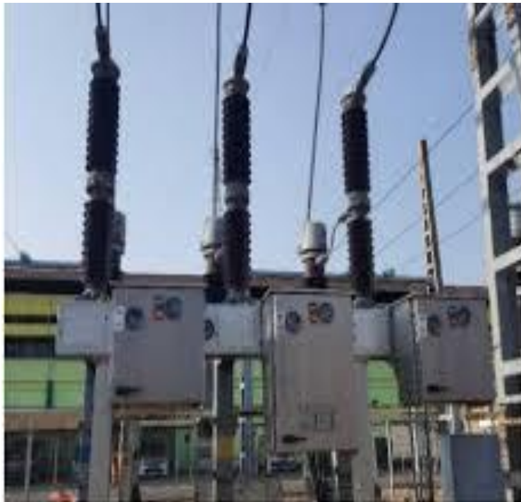
Gambar 2.3 Circuit Breaker (PMT)
