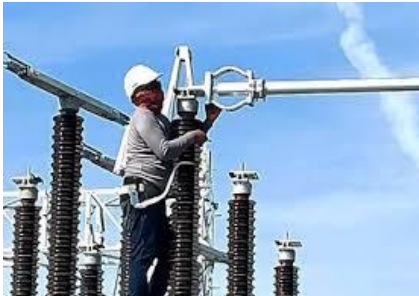
Gambar 2.8 Lightning Arrester
