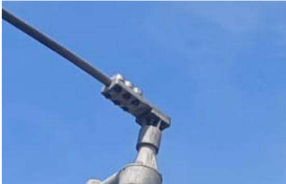
Gambar. 2.2 Sambungan Clamp PMS Bus[4]
