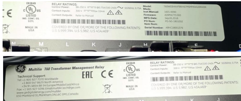
Gambar 3.4 Nameplate Relai Diferensial Merk GE Tipe T60
