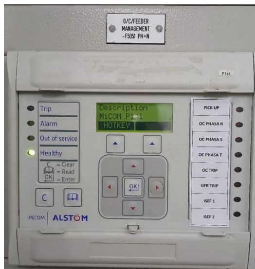
Gambar 2.4 Relai OCR/GFR 150kV
