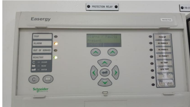
Gambar 2.5 Relai OCR/GFR 20kV
