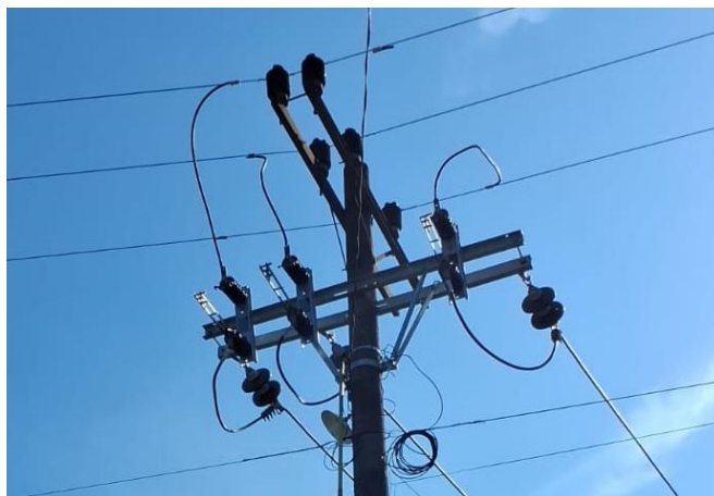
Gambar 2.10. Gambar disconennection swicth/DS )
