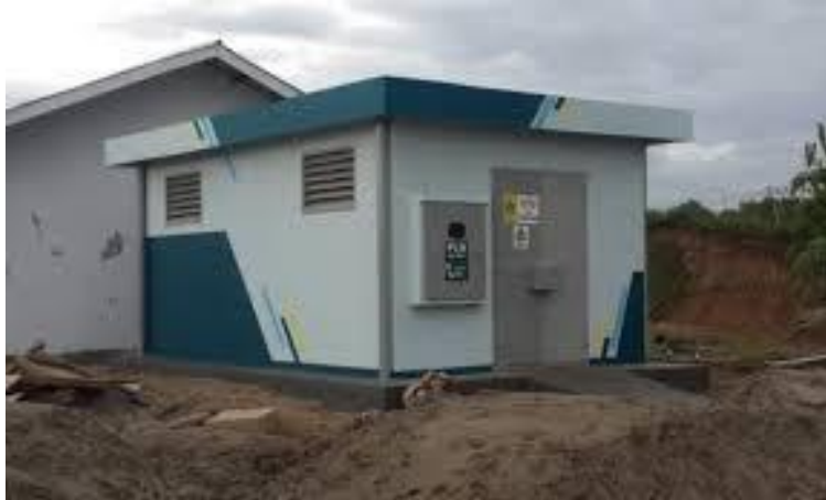
Gambar 2. 5. Gardu Beton
