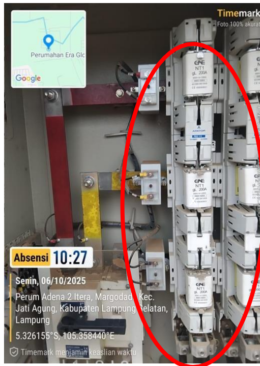
Gambar 2. 12. Fuse Rail
