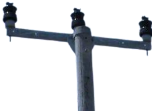
Gambar 6. Travers (Cross Arm)
