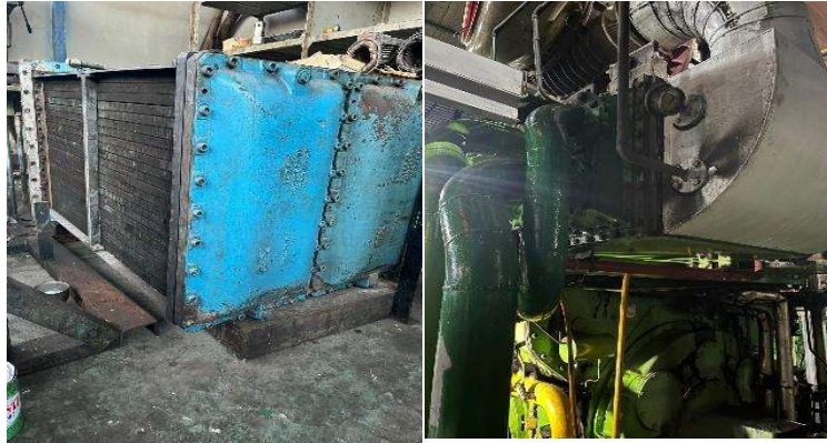
Gambar 2.18. Intercooler
