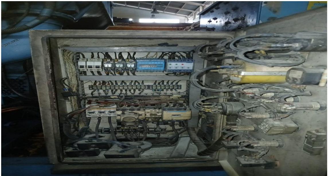
Gambar 2.17 Sistem Pengendalian & Pengaman ( Governor System )
