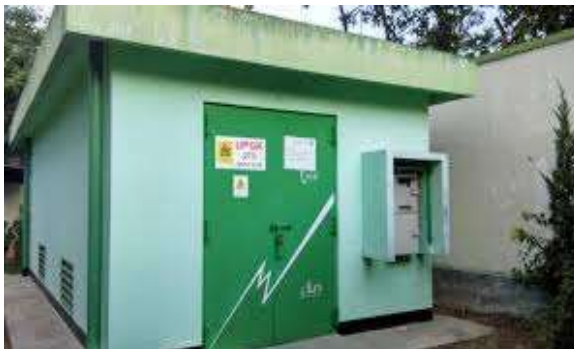
Gambar 2. 3 Gardu Beton
