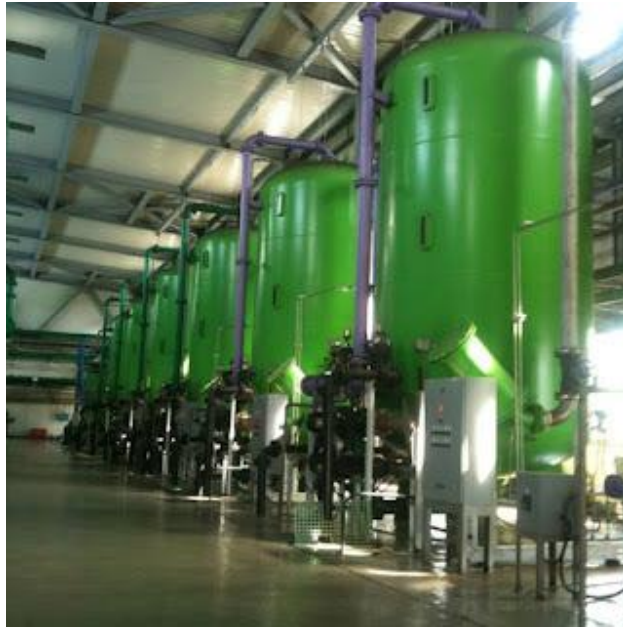
Gambar 2.12 Demineralizer Plant
