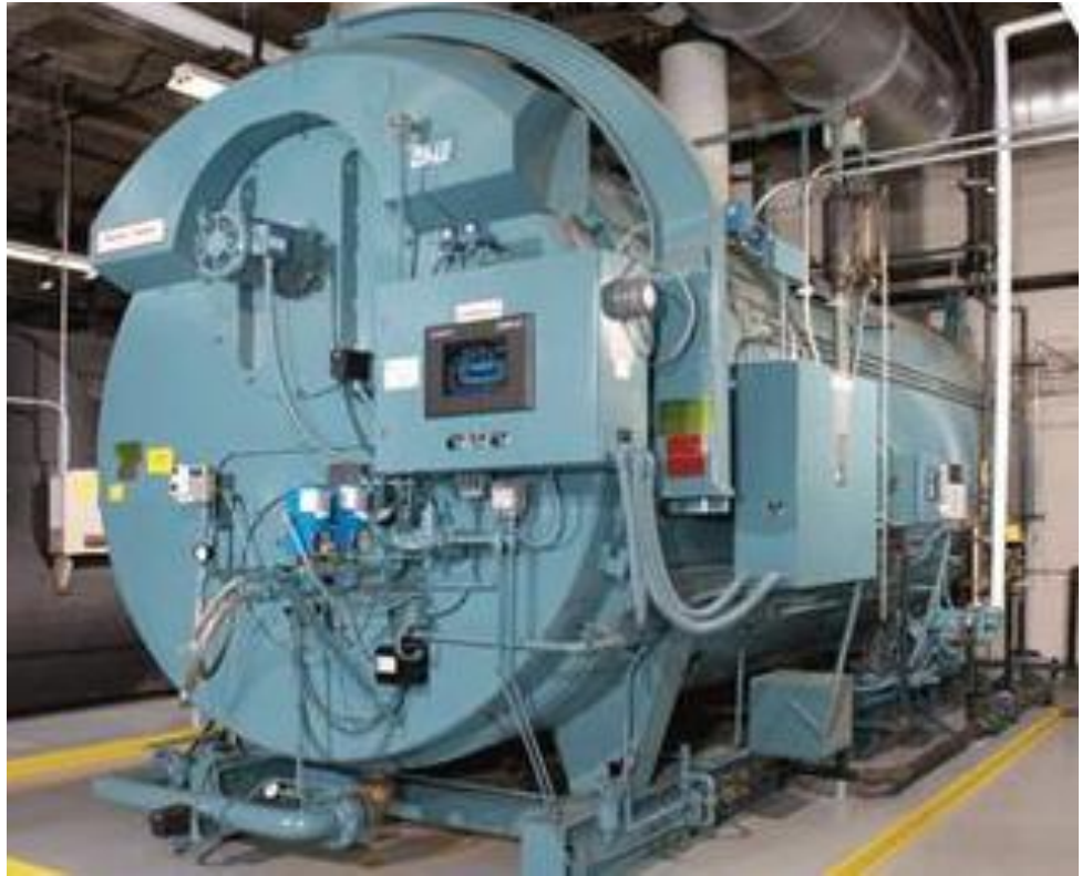
Gambar 2.7 Auxiliary Boiler
