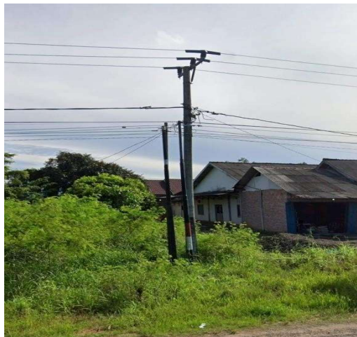
Gambar 2. 1 Tiang Beton 12dAN
