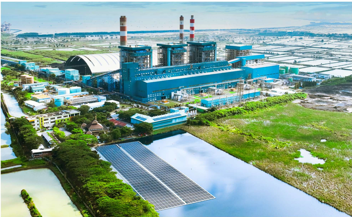
Gambar 2.2 Floating solar PV 1 MWp di area Ash Pond PLTU Banten 3 Lontar
