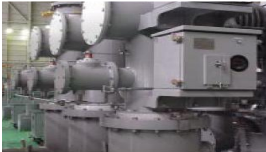
..... Earthing Switch with Motor Operating Box .....
