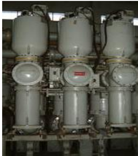
Gambar 2.4: Kompartemen Trafo tegangan (model busbar 1 enclosure – 1 phase)
