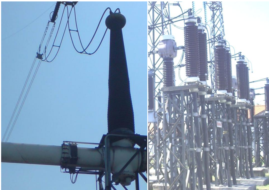
Gambar 2.7: Terminasi/outdoor bushing (model busbar 1 enclosure – 1 phase)
