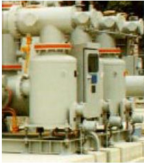
Gambar 2.5: Kompartemen LA (model busbar 1 enclosure – 1 phase)
