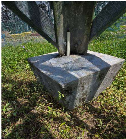
Gambar 2. 4 Pondasi Tower SUTT
