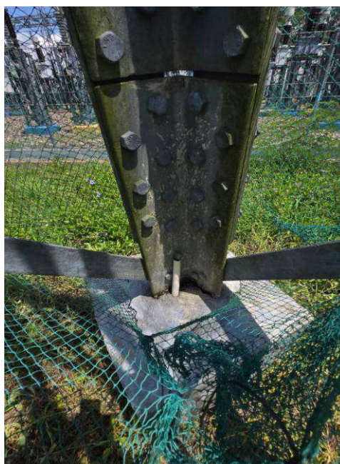
Gambar 2. 5 Stub SUTT
